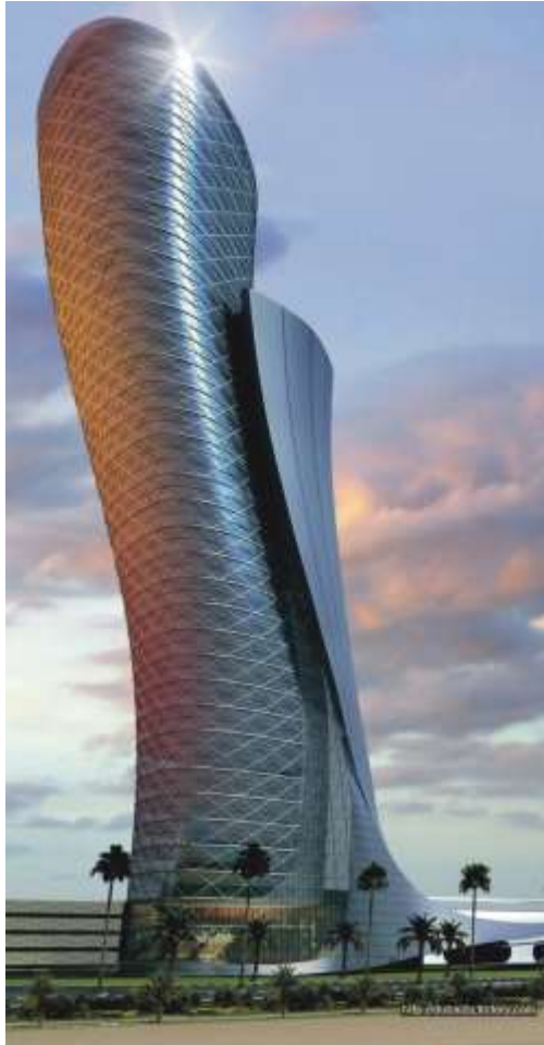
ADNEC Feature Tower | Abu Dhabi
